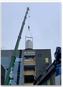
Larger pieces of the plant were removed by crane, requiring the removal of roofing and walls.
