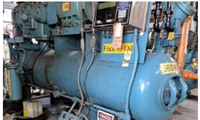
Frick Model RDB316, 200 H.P. Ammonia Rotary Screw Compressor
